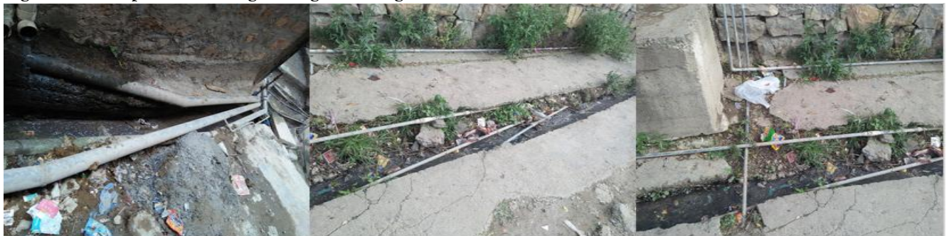
Fig. 2 Water Pipelines Passing through Sewerage
